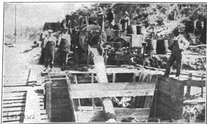
FIG. 5. CONCRETE-MIXING PLANT, WITH STEEL PIPE CHUTE TO FORMS FOR PEDESTALS
